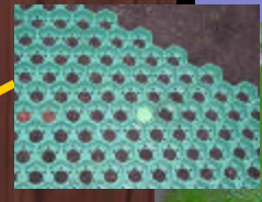
The Golpla Structural grass filled with top soil and seeded
